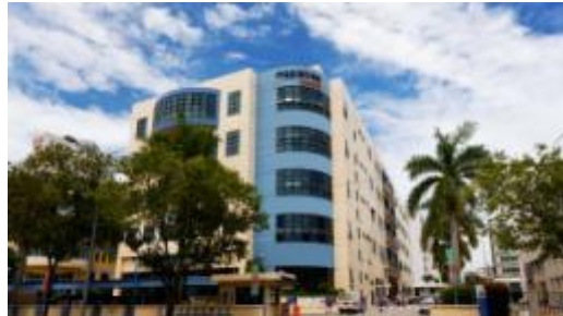
Light Industrial Buildings
